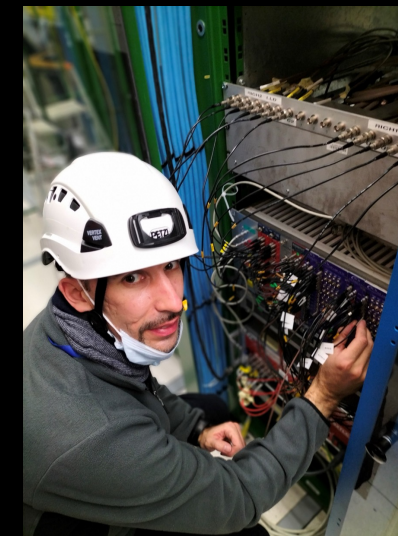
LLD installation at CERN
