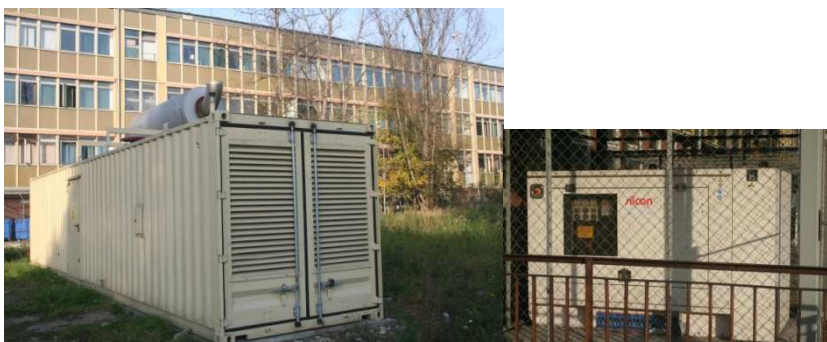
Power supply - generators 1 MW (diesel) and 50 KW
