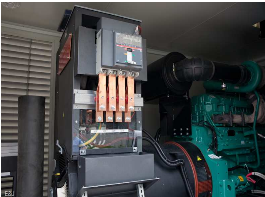
← TASK - diesel generator 0.9 MW
