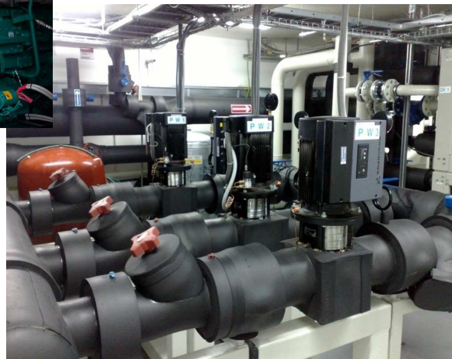
ICM – ice water cooling system → 1.3 MW
