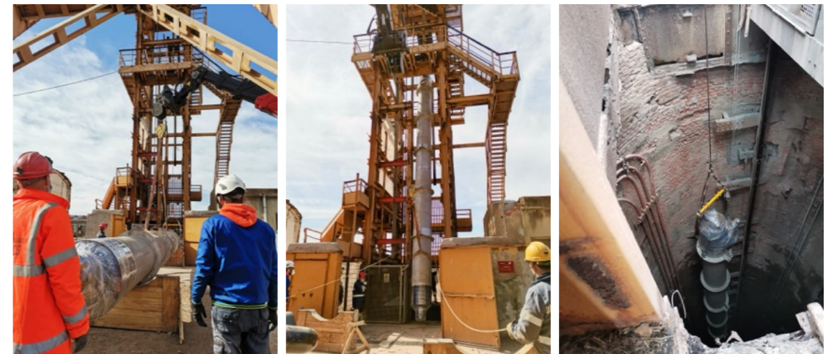
Test installation of the module
