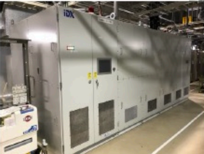
New horn PS for 320 kA/1Hz operation
