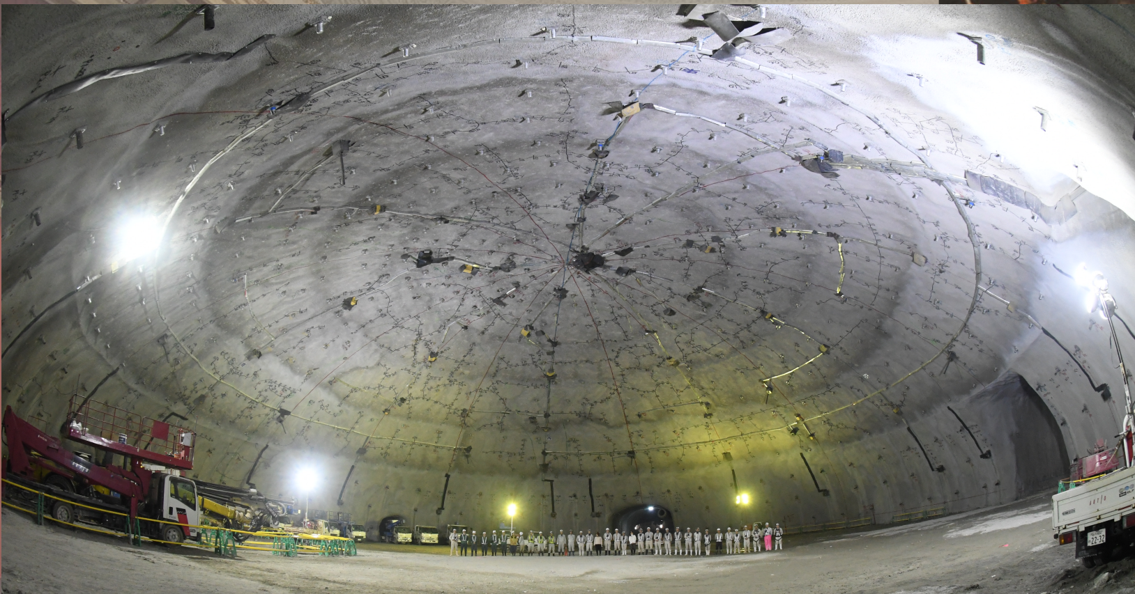
Oct. 3, 2023 Completion of the dome (dia. 69 m, height 21 m, ~1 Super-K)
