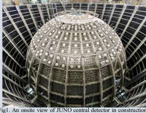
Fig1. An onsite view of JUNO central detector in construction
