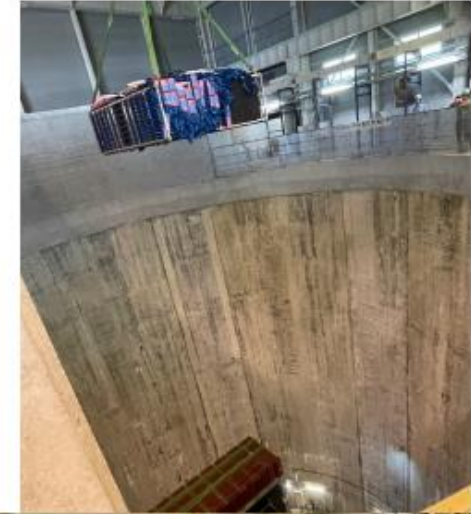
Super-FGD installation (October 2023)
