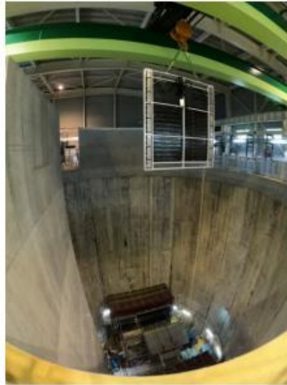
TOF installation (July 2023)
