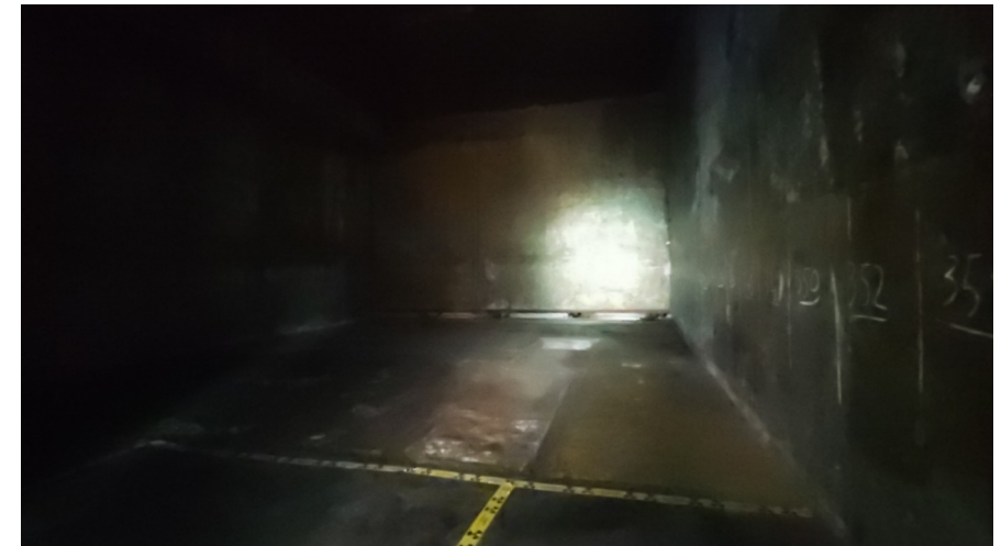
Installation in complicated environment
