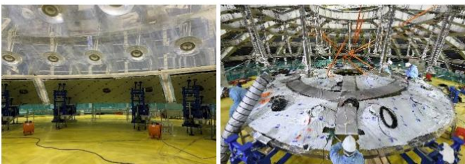
⑤ unloading, sanding, polishing, cleaning, filming
