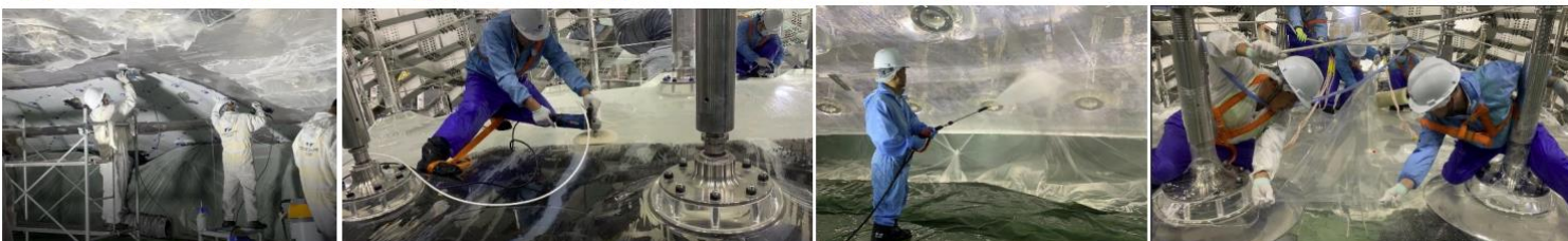
⑤ unloading, sanding, polishing, cleaning, filming
