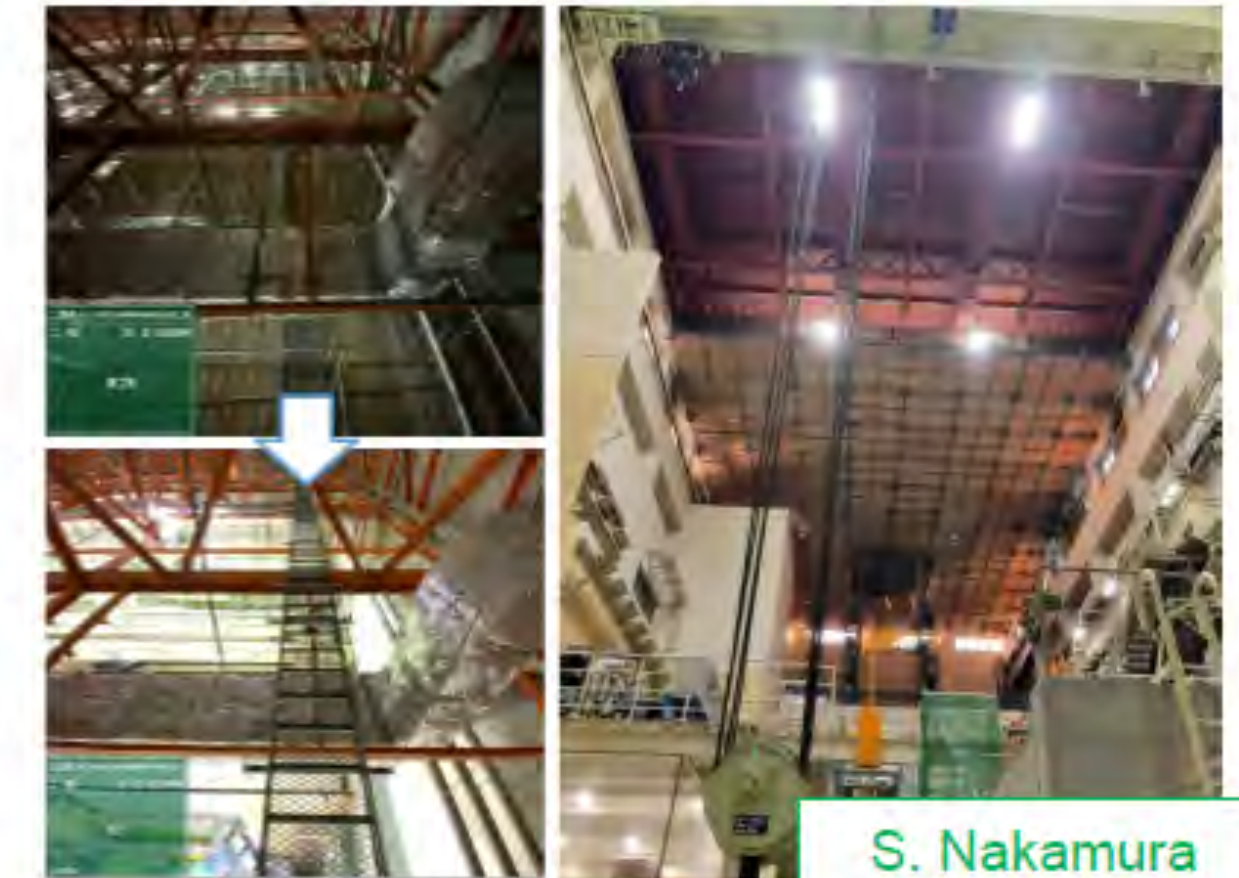
Ceiling aseismic reinforcing work
