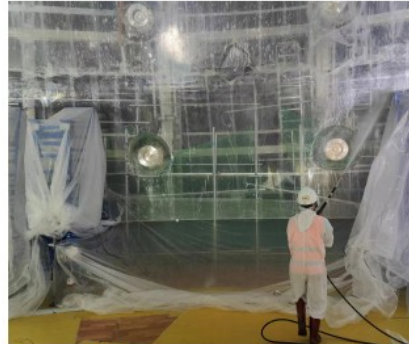
Cleaning inner surface
