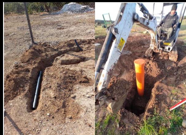
Three magnetometers are (three direction N-S, E-W and vertical) located at the two boreholes
