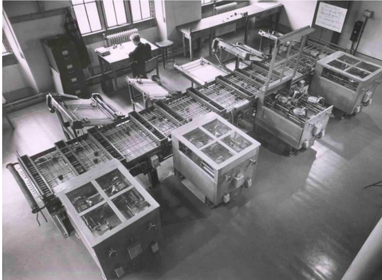
Differential analyzer, 1938 (University of Cambridge)
