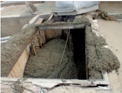
*Concrete poured into the shaft in attempts to stop the crack*
