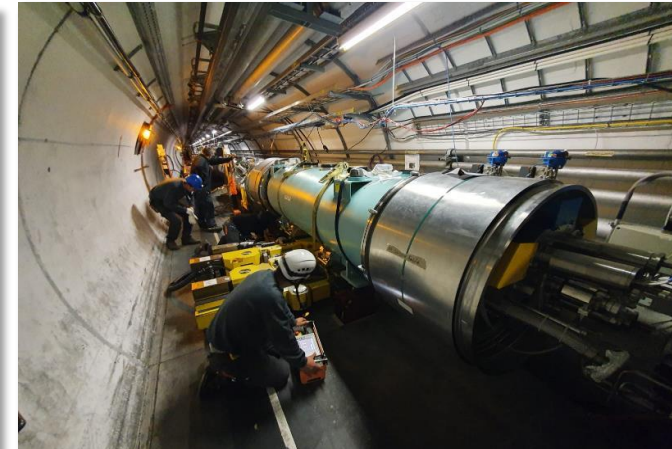
LHC connection cryostat
