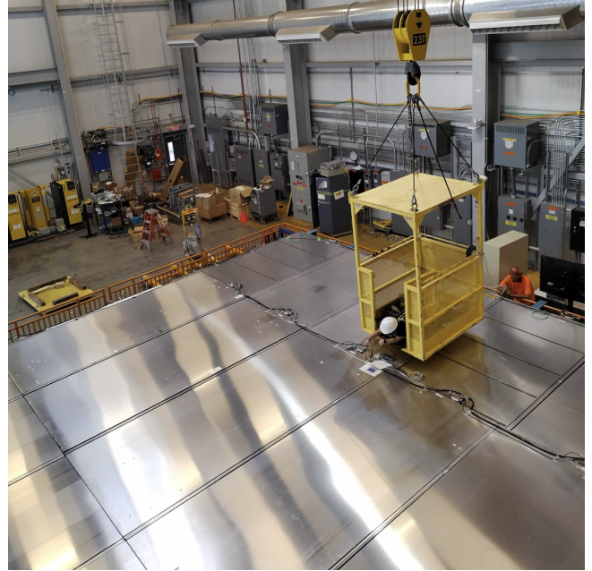
Figure 8: Photo of me working from the basket to ground the modules of the CRT Top High.
