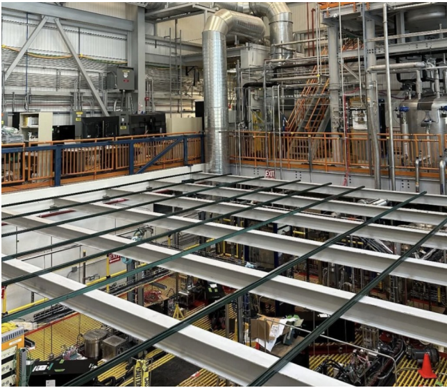
Figure 7: Photo of the initial state of the detector before the installation of the Top Low and Top High layers of the Cosmic Ray Tagger.
