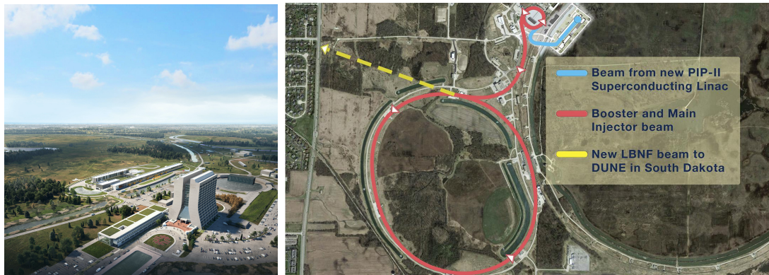
Figure 1.2: The new complex of buildings, located near Fermilab’s Wilson Hall, will host PIP-II particle accelerator. It will be the new heart of the Fermilab accelerator complex, that comprises also the existing Booster ring and Main Injector-Recycler.
