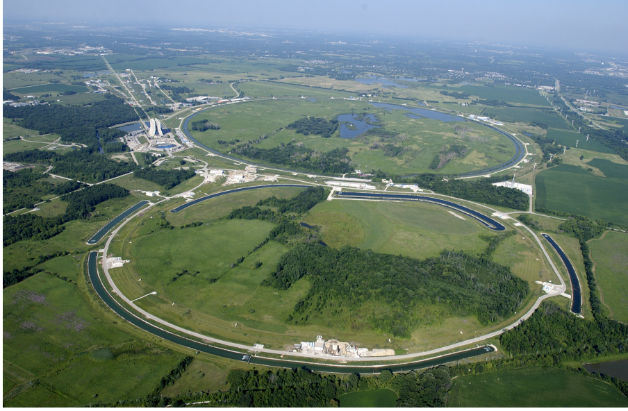
Figure 1.3: Aerial view of Fermi National Accelerator Laboratory. The 3.2 km circumference Main Injector tunnel is visible in the foreground, the Tevatron tunnel is visible in the background. The High Rise is in the top left corner. The Tevatron has been the most "powerful" particle accelerator for many years before the turning on of the Large Hadron Collider (LHC) at CERN in Geneva.
