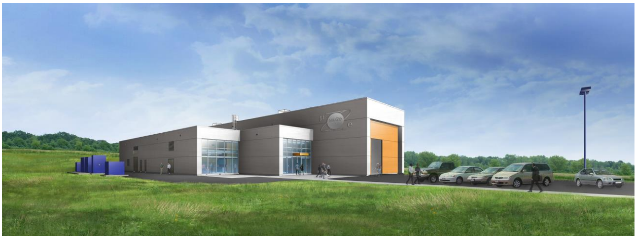
Figure 2.2 - Depiction of the above-grade portion of the Mu2e facility. (L. Bartoszek et al.)
