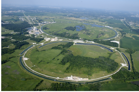
Fig. 1.3: Aerial view of the Fermi National Accelerator Laboratory. The 3.2 km circumference Main Injector tunnel is visible in the foreground, the Tevatron tunnel is visible in the background. The Mu2e facility is located next to the High Rise. The Tevatron has been the most "powerful" particle accelerator for many years before the turning on of the Large Hadron Collider (LHC) at CERN in Geneva.
