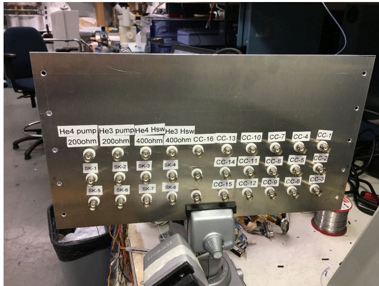
Figure 3.0.4: View of the BNC connectors hosted on one side of the box.
