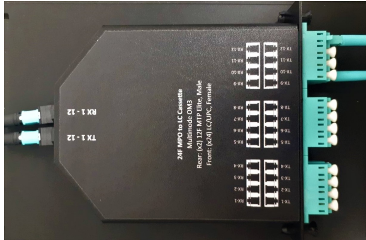
Figure 5.5: Fiber cassette: it is the optical splitter from 12(x2) MTP Male to 24 LC/UPC Female.
