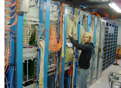
Fiber cabling on the readout system
