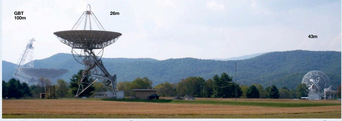
Array is 43m and two 26m antennas arranged roughly in a triangle with 0.8 to 1.5 km baselines.
