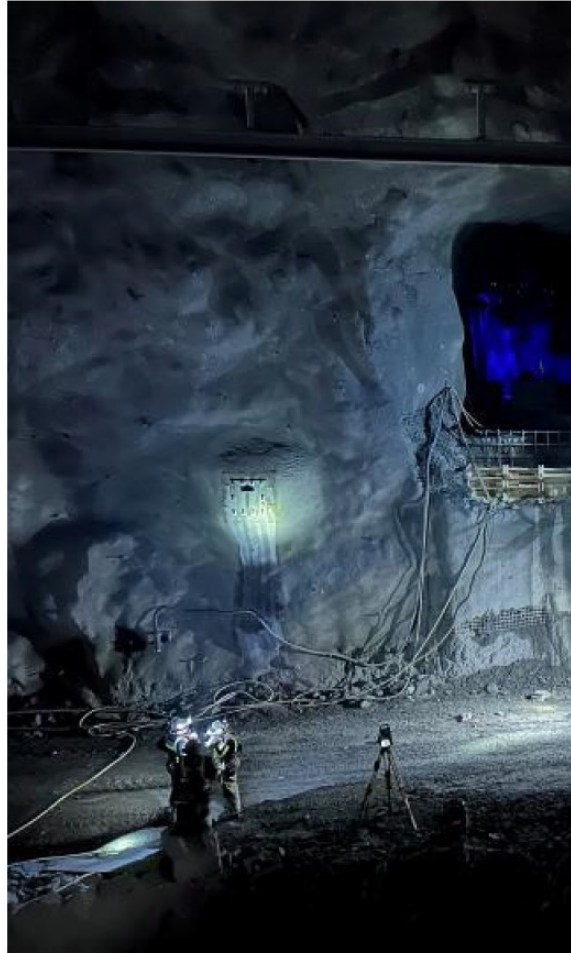
North Cavern –midpoint connection drift
