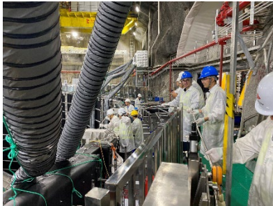
PMT cables deployment
