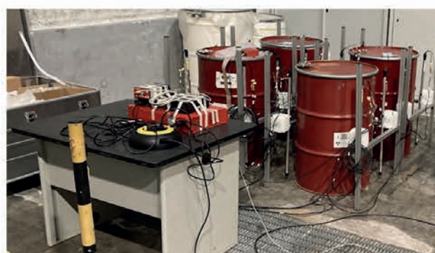
Figure 2. The monitoring system installed around the LLW drums at NUCLECO.
