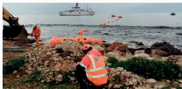
Figure 2: Arrival of the IDMAR cable at the Capo Passero harbour.
