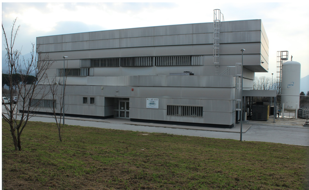
Figure 3- View of the THOR Lab at University of Salerno – Italy.
