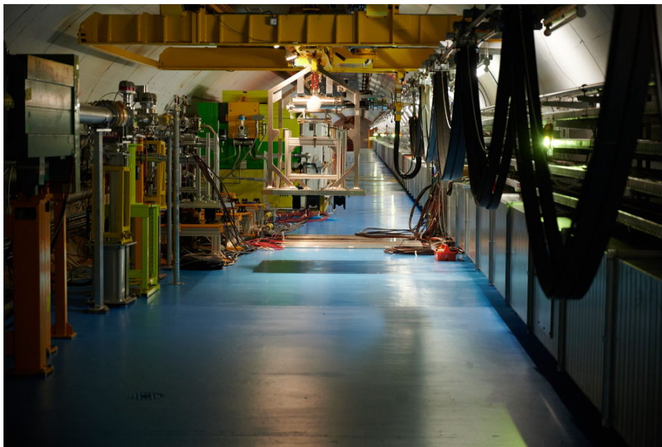
Figure 1- View of the facility during the remote installation of an experiment.
