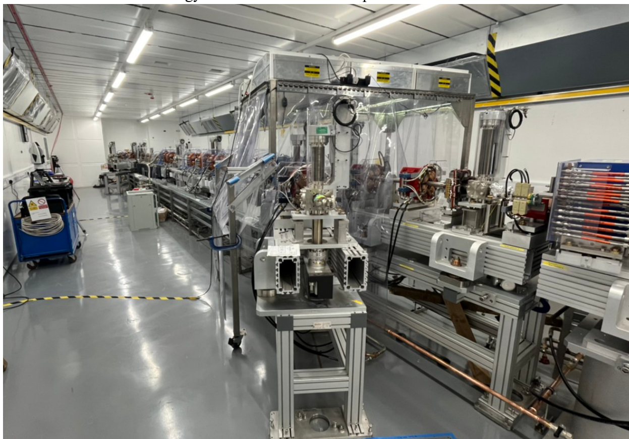
Figure 14- View of the CLARA facility (phase 2 construction).
