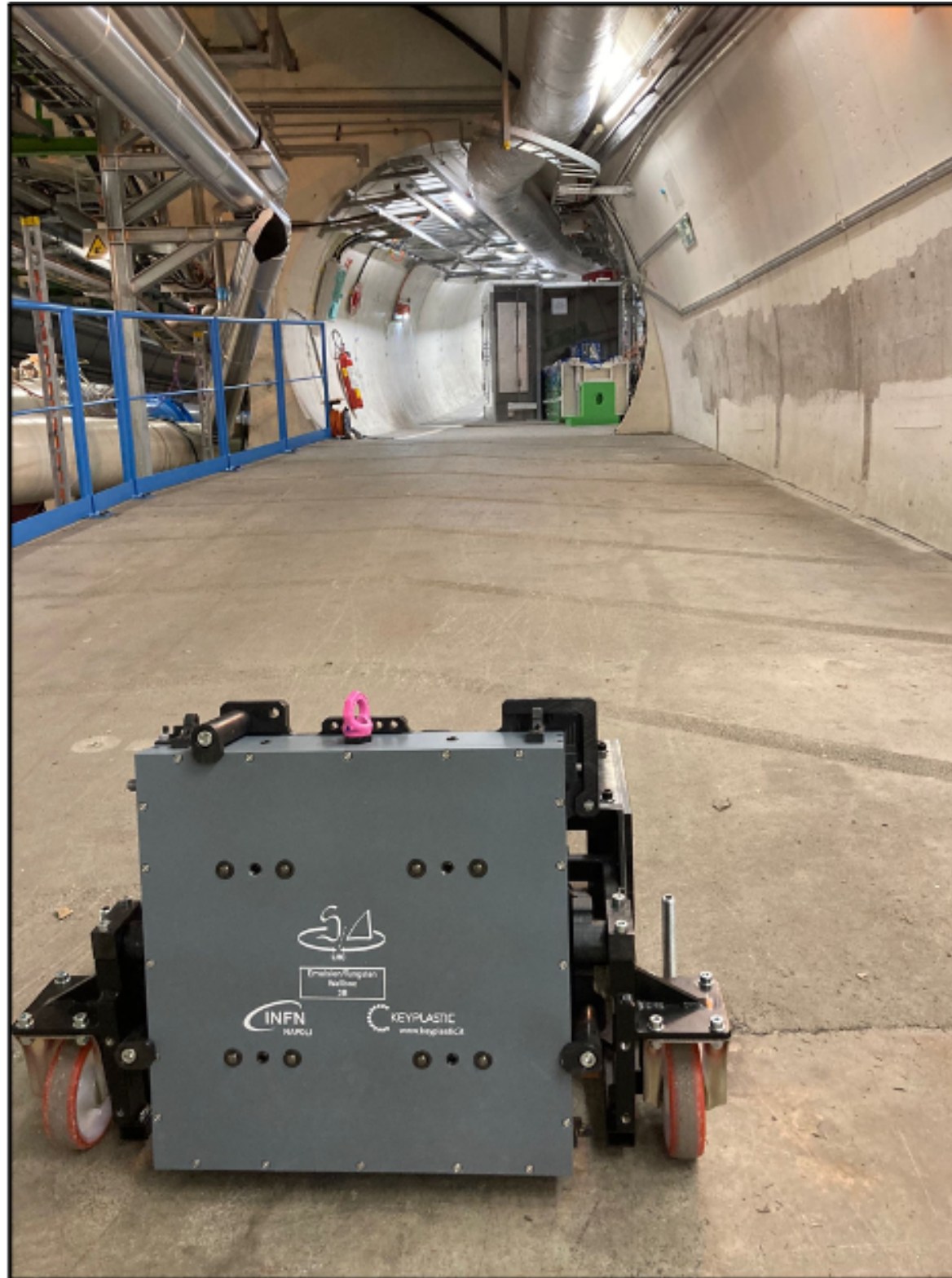
April 7 th - Installation
