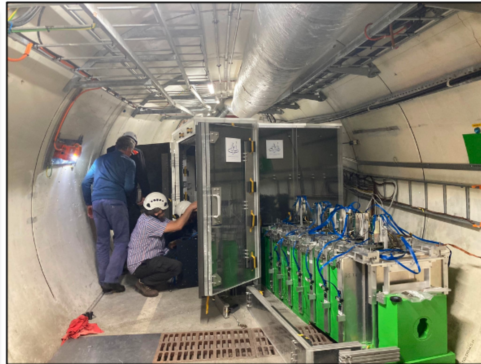
September 13 th – Installation
