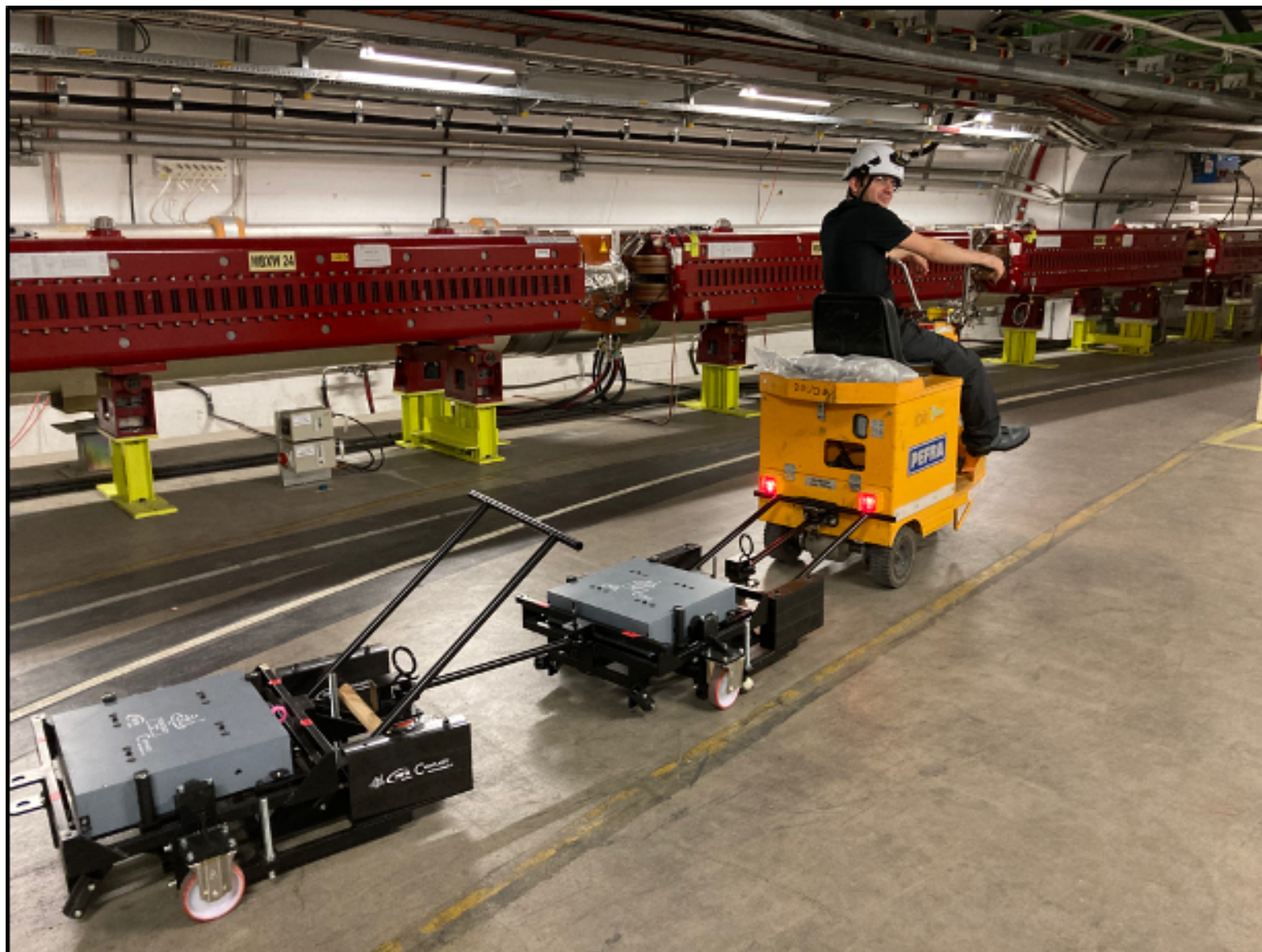
July 26 th - Installation
