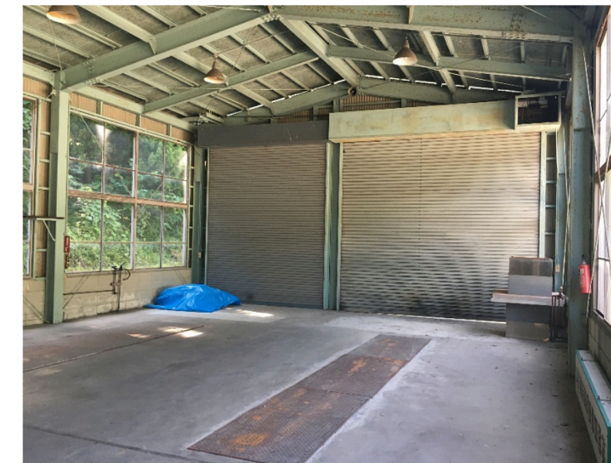
Warehouse #2 (~13m x ~9m = ~117m 2 )
