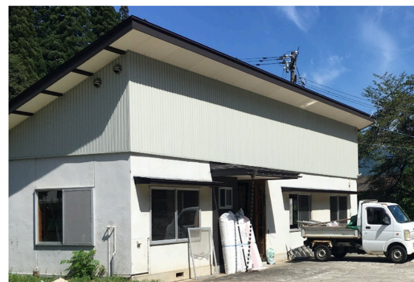
Small office space (under refurbishment)
