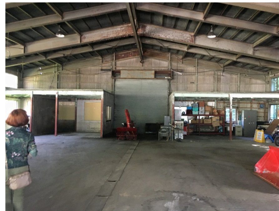
Warehouse #1 (~24m x ~18m = ~432m 2 )
