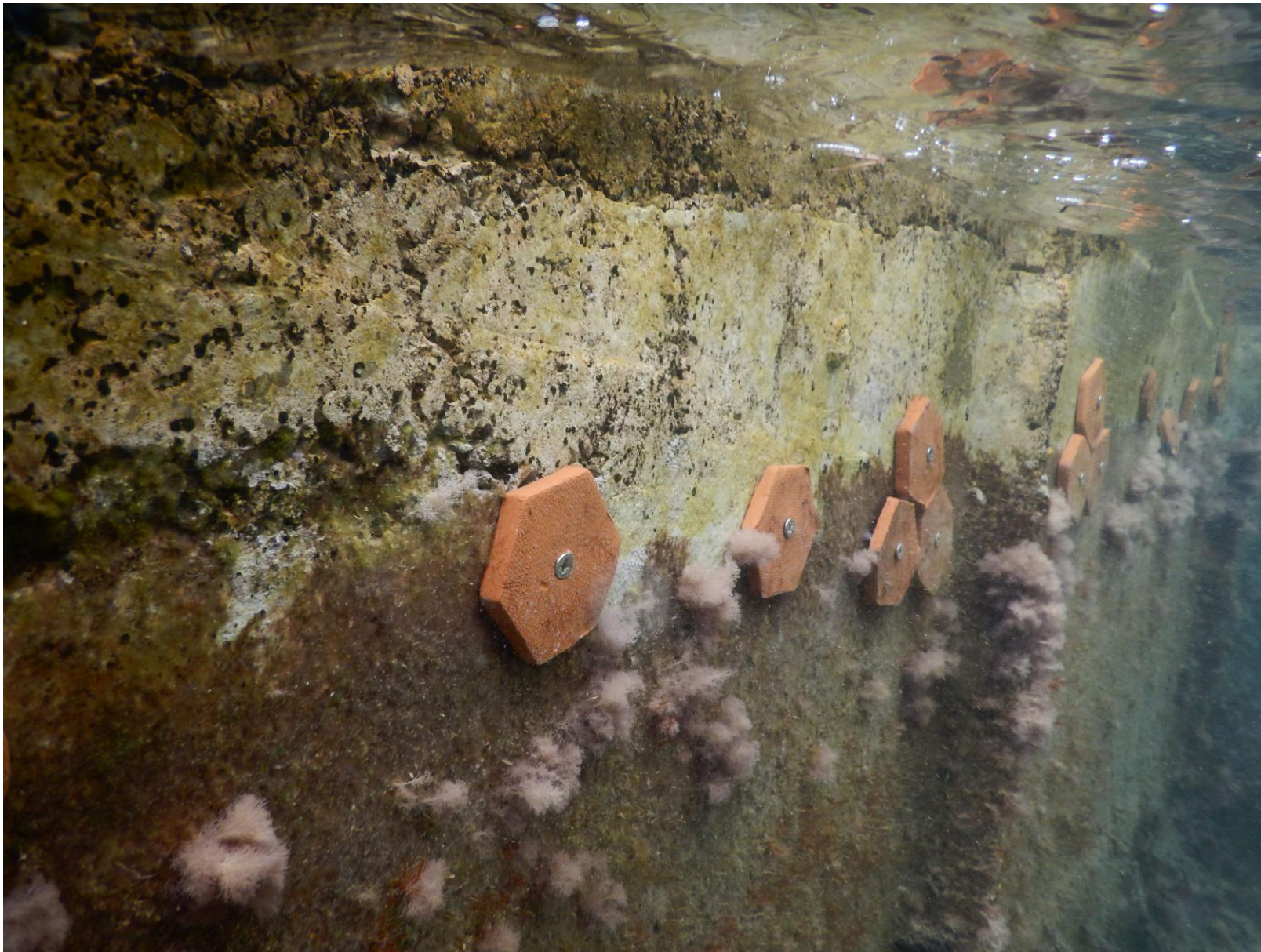
Artificial reef with clay tiles, after last summer's deployment
