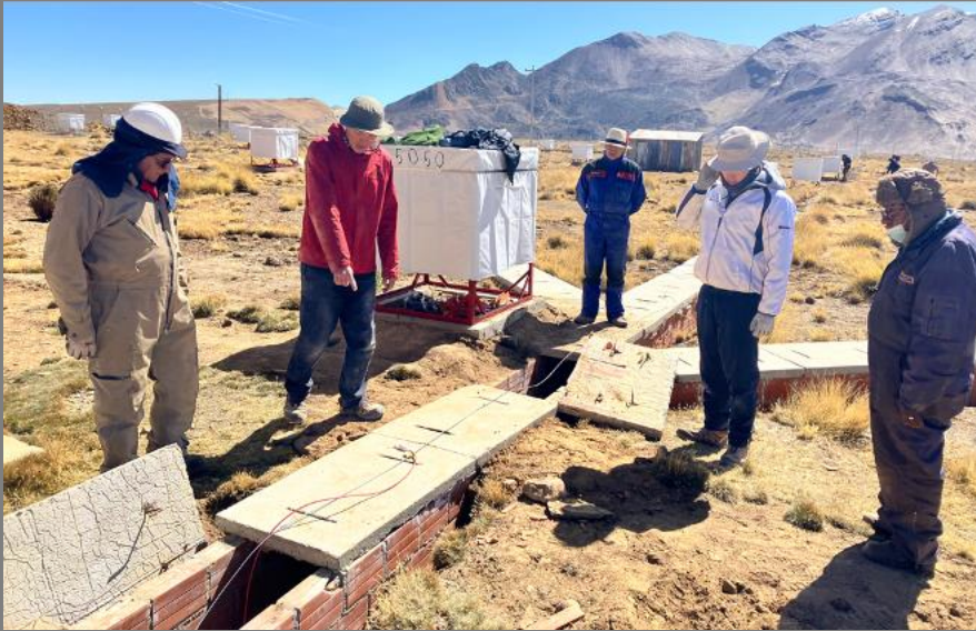
Installation of cables
