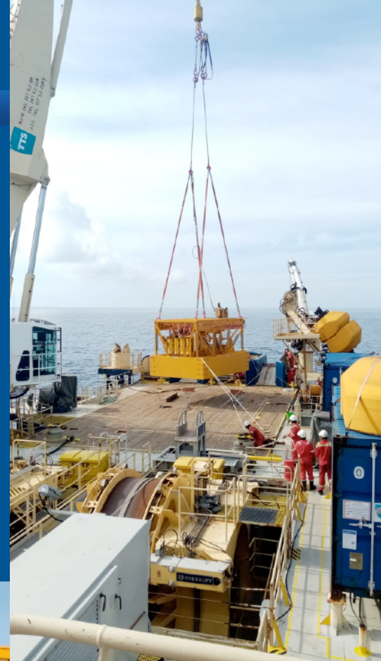
Cable Termination Frame
