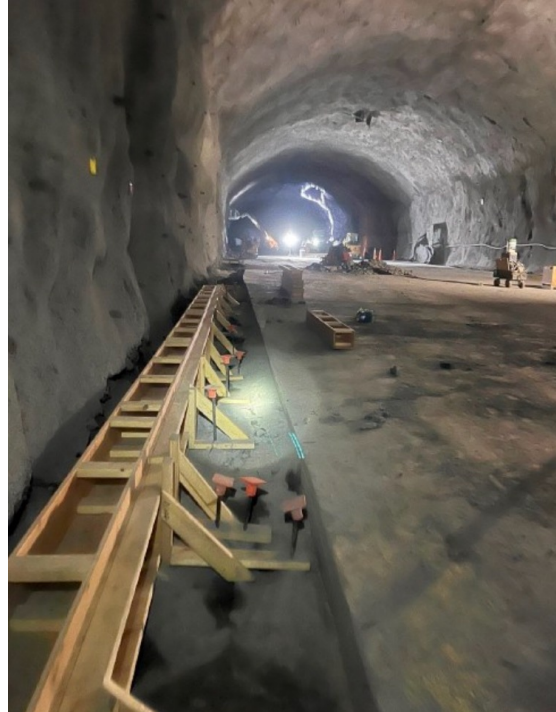
Central utility cavern
