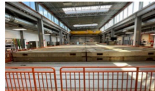
June 7 th 2022: completion of overburden installation
