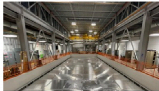
Dec. 2021: completion of CRT installation
