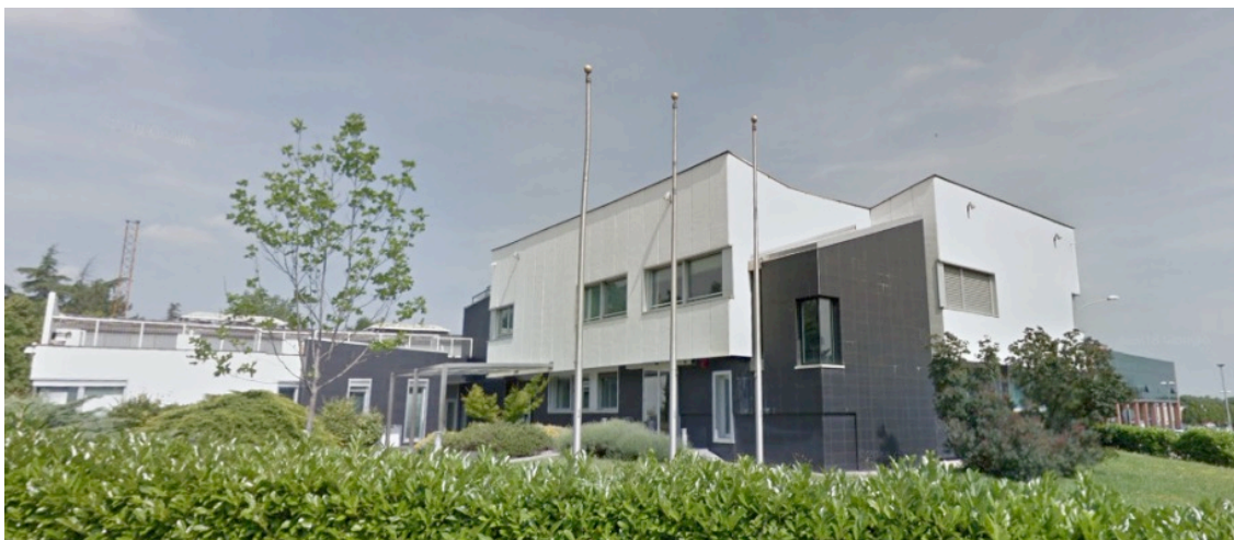
Figure 5 Temporary ICSC building (Bologna)
