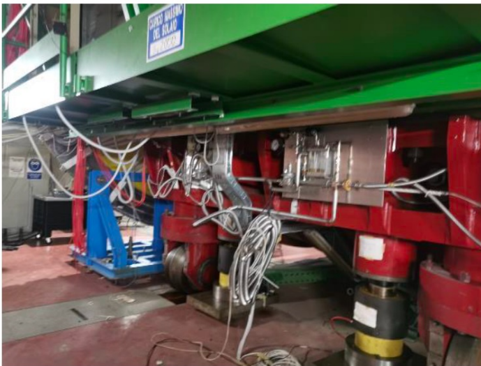
Removal of not reusable instrumentation
