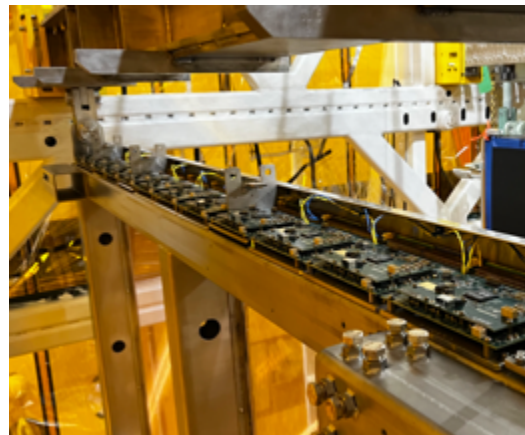
Cold electronics installed (Dec 2021)
