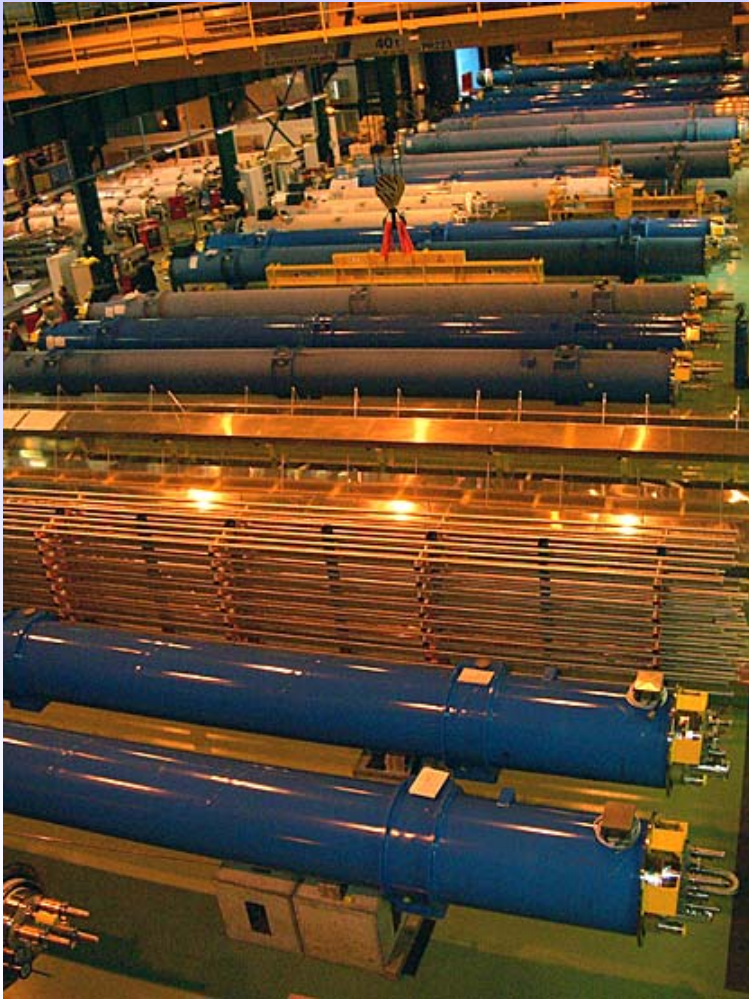
Preparation for installation, Hall SMI2
