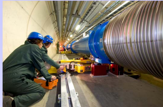
Installation work, underground
