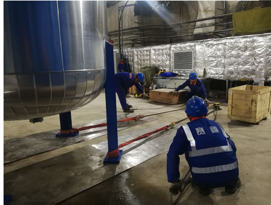
罐体吊立后向两侧移动 move aside after lifting
