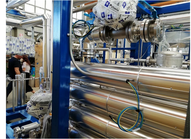
Cabling of valves and instruments
