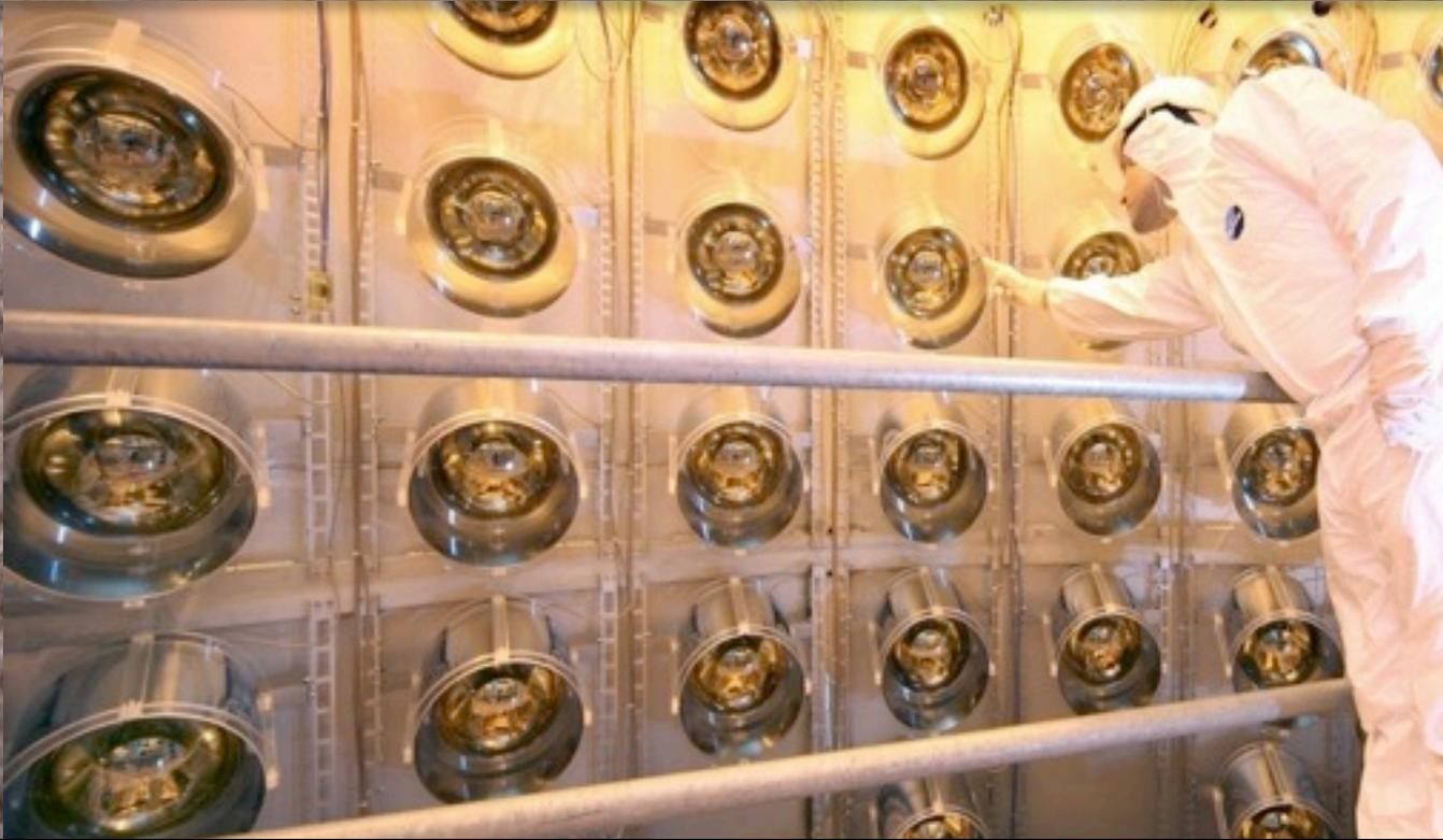
Inner-Detector  $\Rightarrow$  PMT installation
