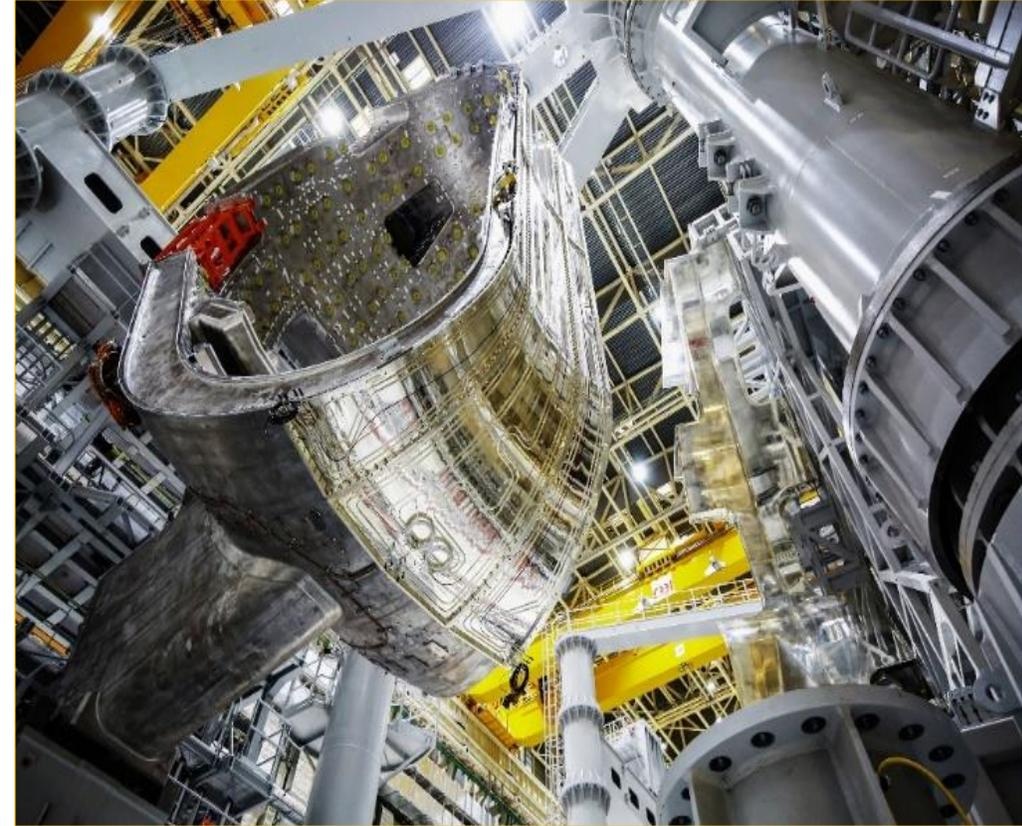
« Sub-assemblies » are the building bricks of the Tokamak's torus. They comprise one 40° vacuum vessel sector, two toroidal field coils and the corresponding thermal shield panels, and weigh in excess of 1,250 tonnes.
