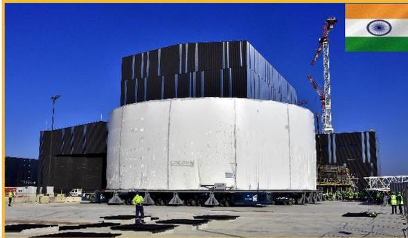
Cryostat Lower Cylinder
