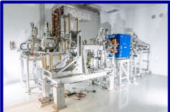
Target Ion Source Complex
