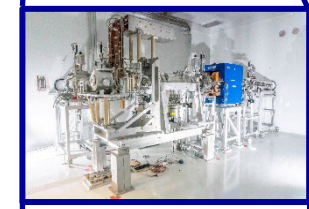
Target Ion Source Complex
