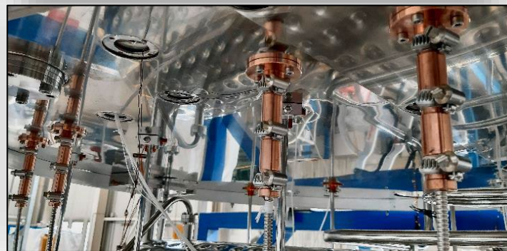
New thermal joints
