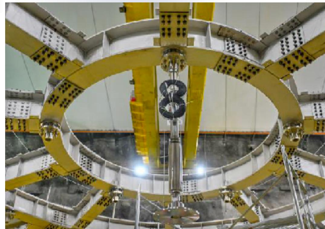
Assembly precision must be < 3 mm to maximize PMT number
