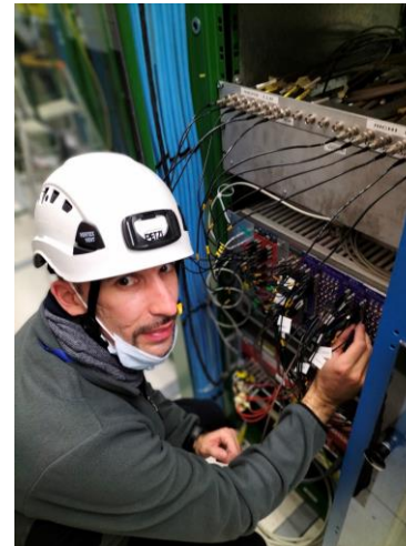
LLD installation at CERN
