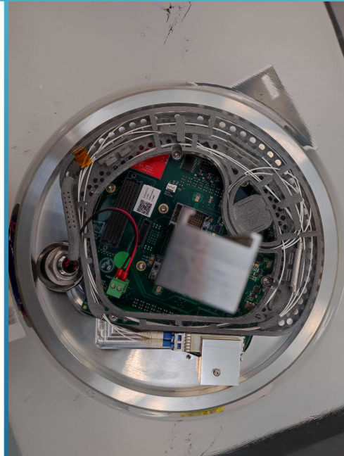
CLB and electronics installed
