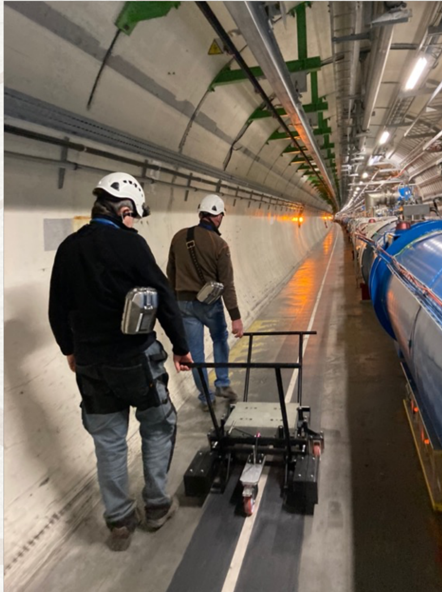
In the LHC tunnel
