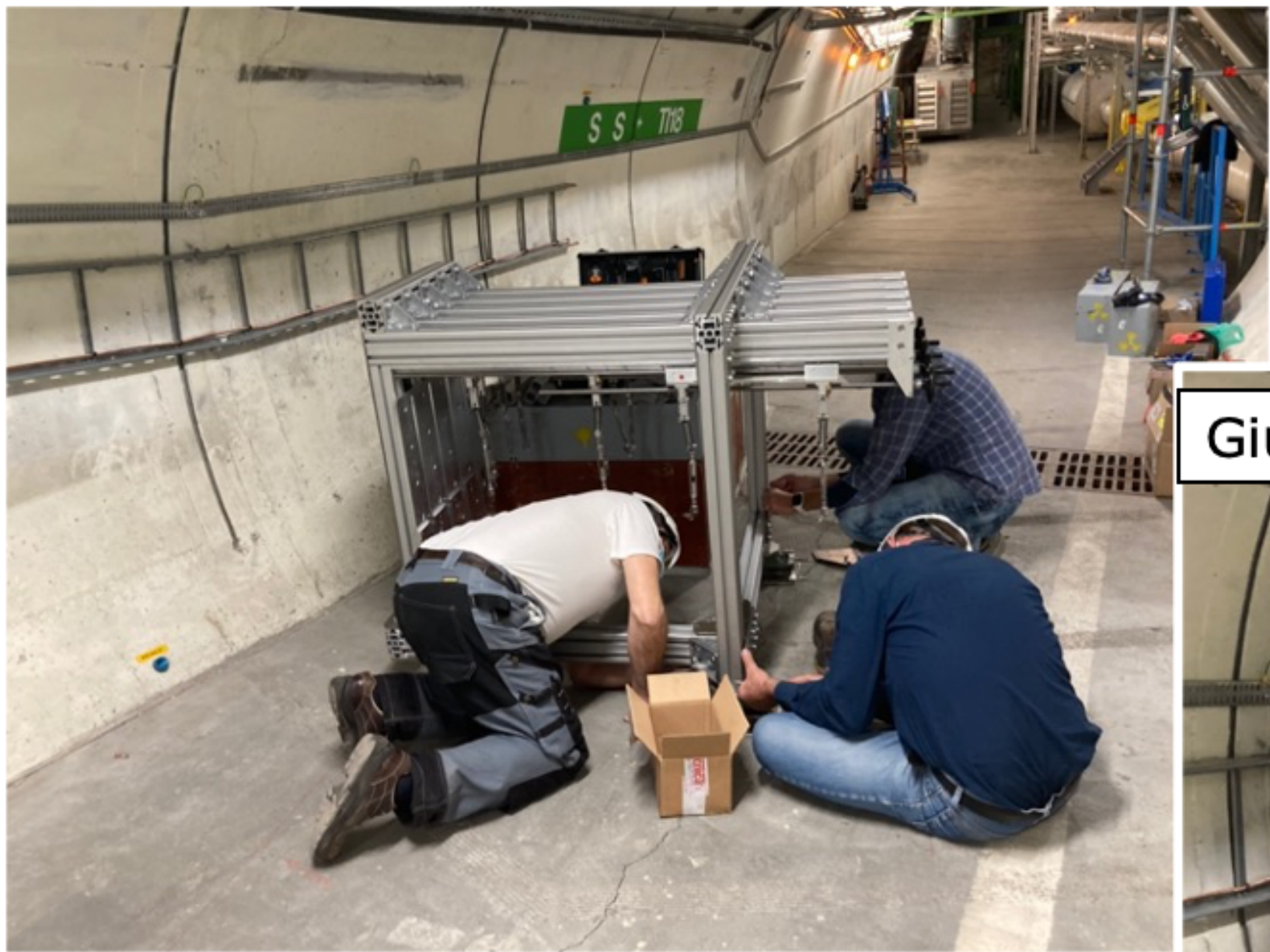
Target structure installation
