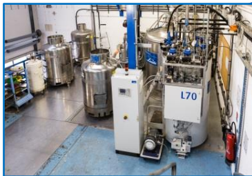
Helium gas recovery and compression hall helium gas compression associated with a helium liquefier
