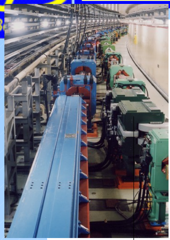
Replace short dipoles with longer ones (LER)
